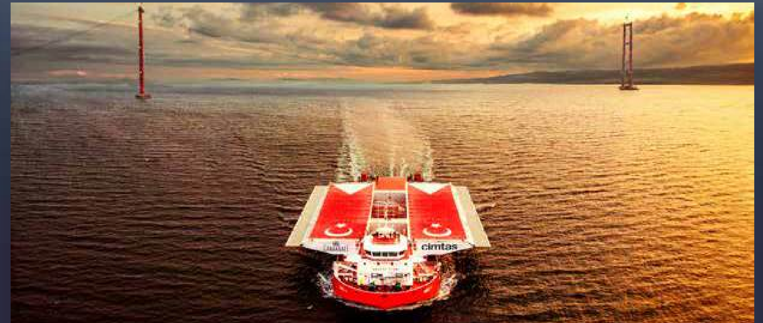
1915 ÇANAKKALE SUSPENSION BRIDGE
