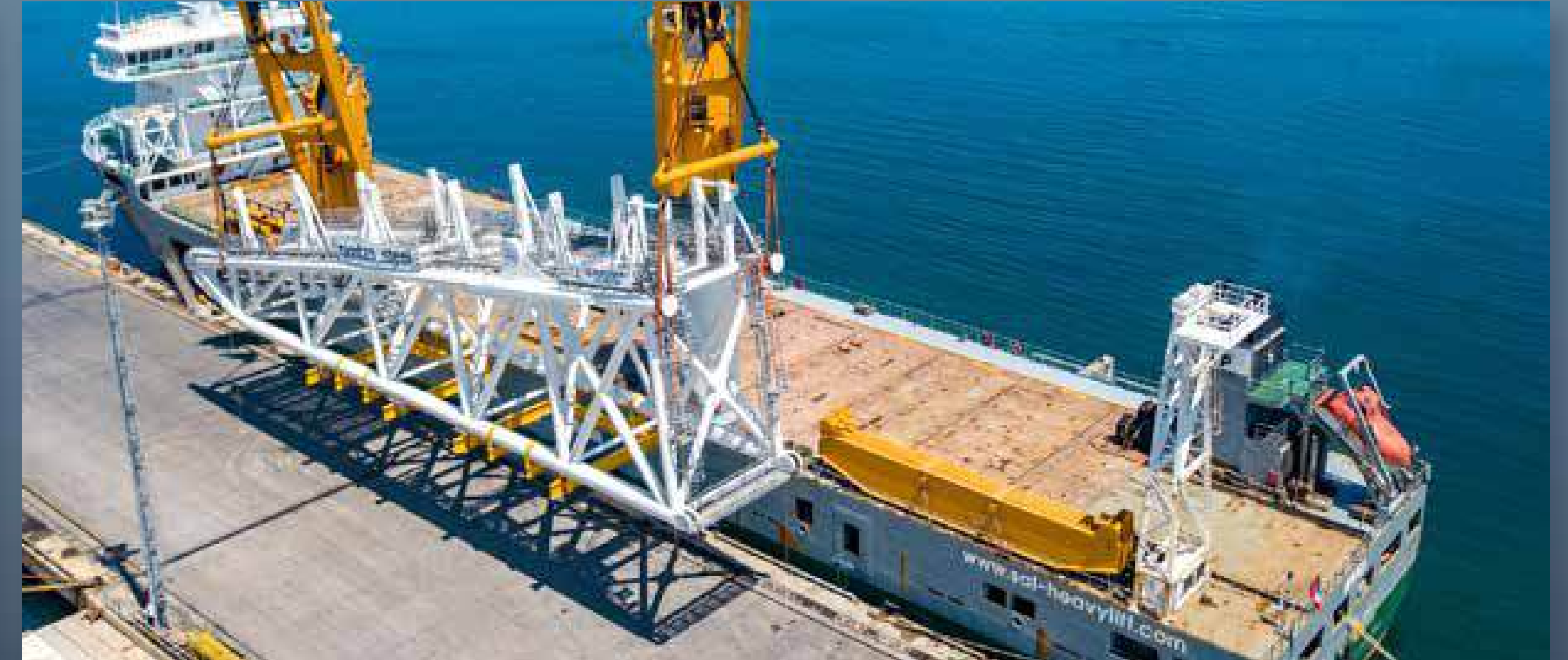
STINGER SECTION PROJECT
