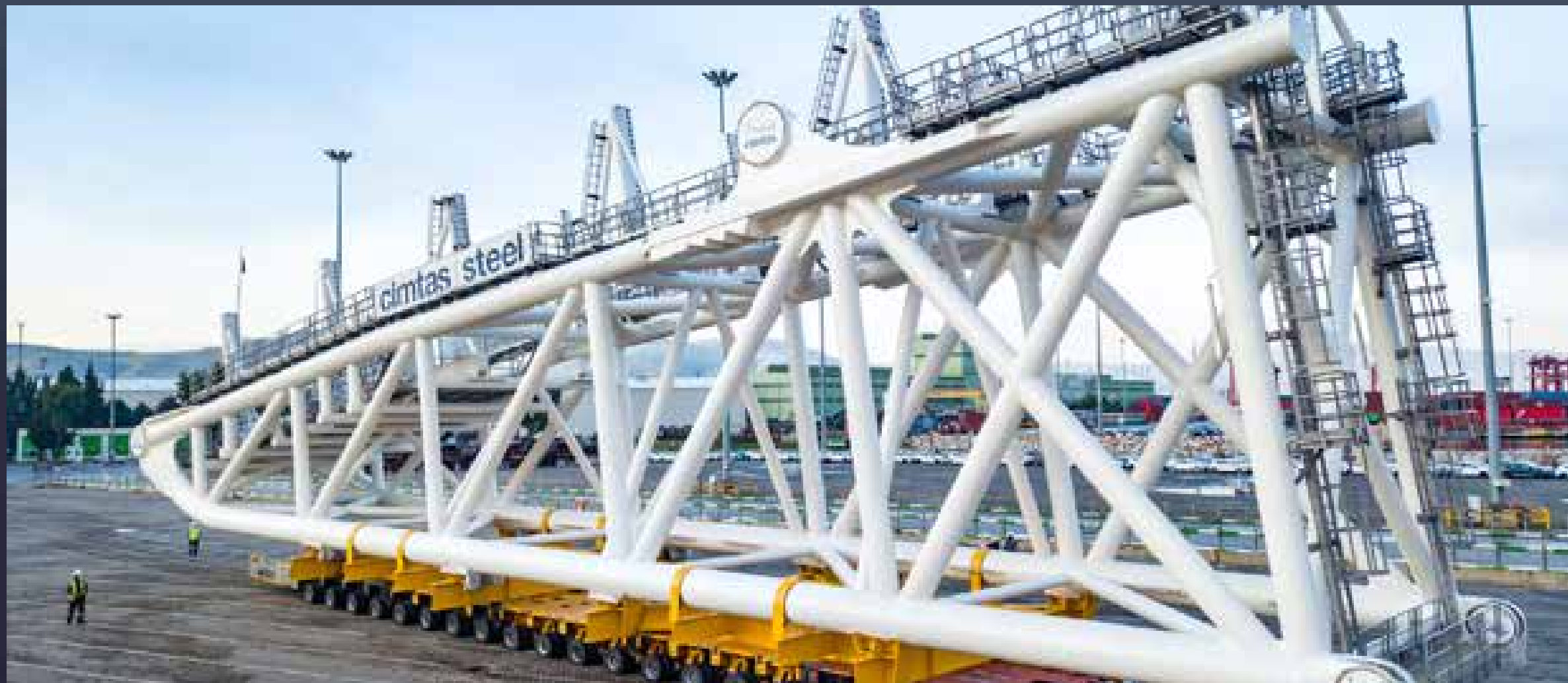
STINGER SECTION PROJECT
