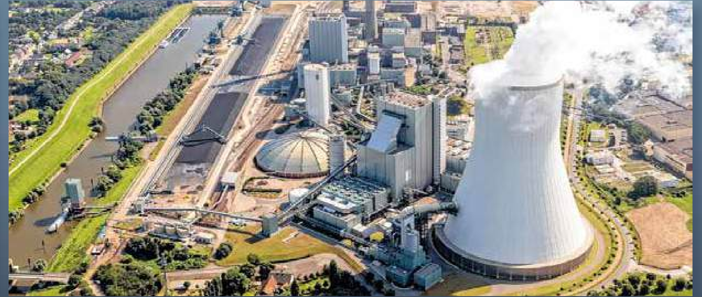
WALSUM COAL FIRED POWER PLANT 800 MW
